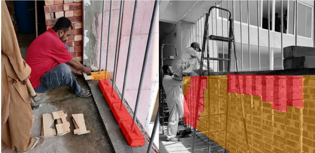
Fig. 11. Conventional brick masonry using custom wooden jigs based on colour codes.
