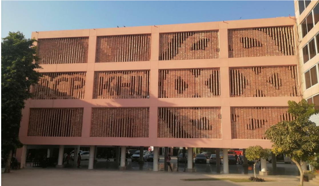
Fig. 12. Southern façade of the Brick Screen at ACPKHI, Karachi, Pakistan.
